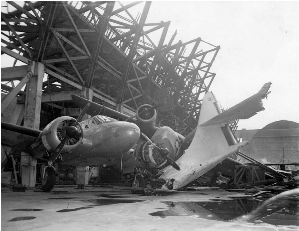
Figure 2. Devastation of Richmond NAS following the hurricane and fire of September 15 th 1945 (Freeman 2017).
